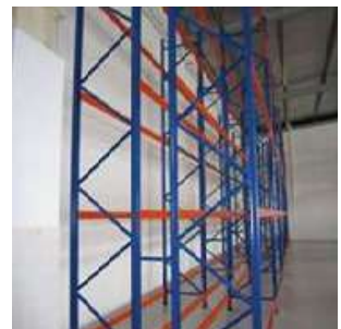
APR: Adjustable Pallet Racking – Double Deep LIFO High storage density, space utilisation increases. However, additional height clearances may be required. Suitable for low stock rotation or low throughput.
